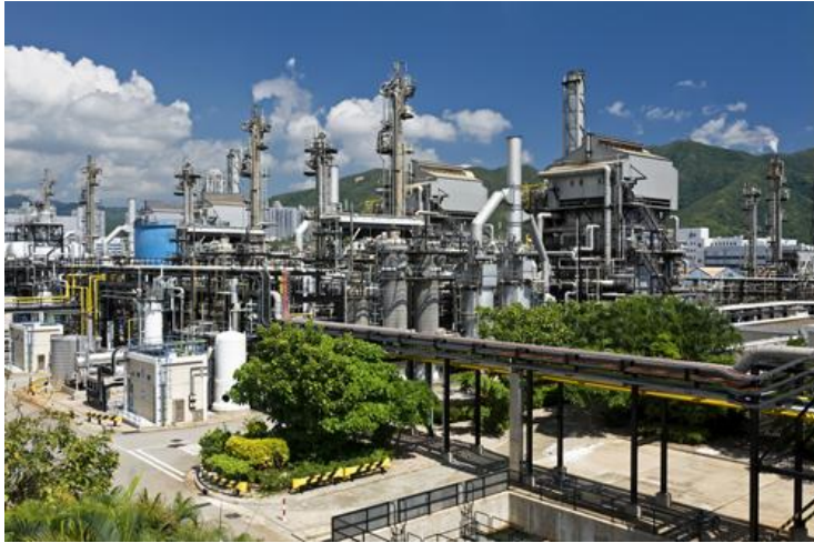
Figure 6.3 Tai Po Gas Production Plant Source: Environment Bureau
