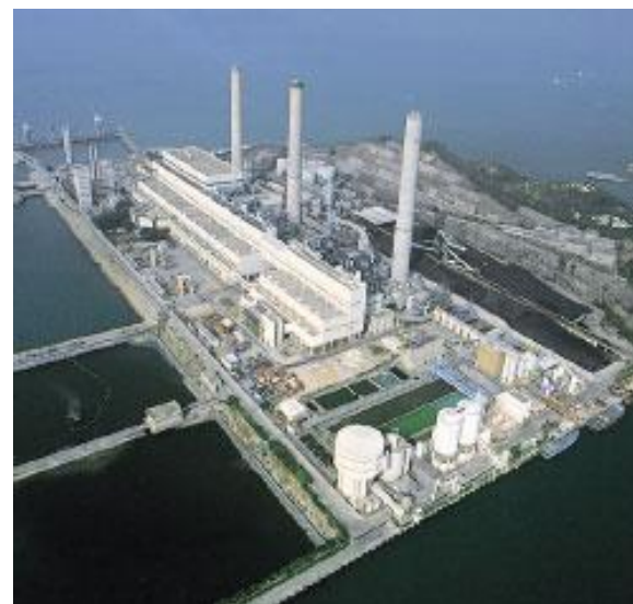
Figure 6.1 Lamma Power Station Source: Environmental Protection Department
