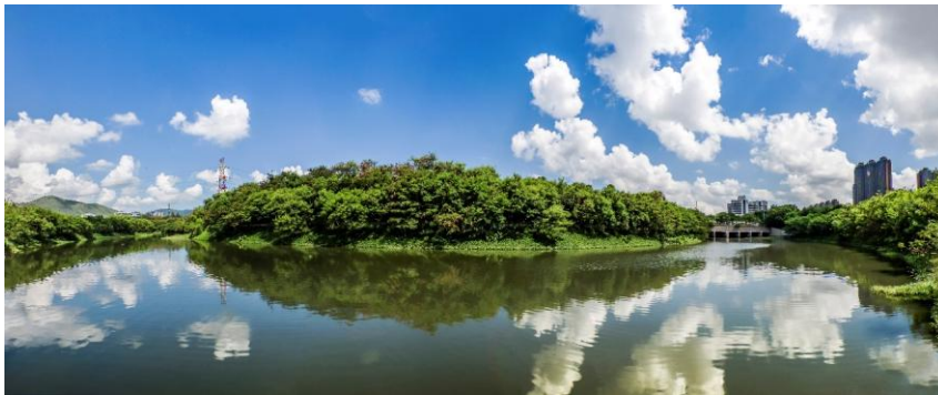
Figure 4.1 Yuen Long Bypass Floodway is constructed to improve drainage capacity of Yuen Long Town
