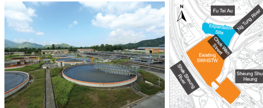
Figure 3.4 Existing Shek Wu Hui Sewage Treatment Works (Left) Source: Drainage Services Department
