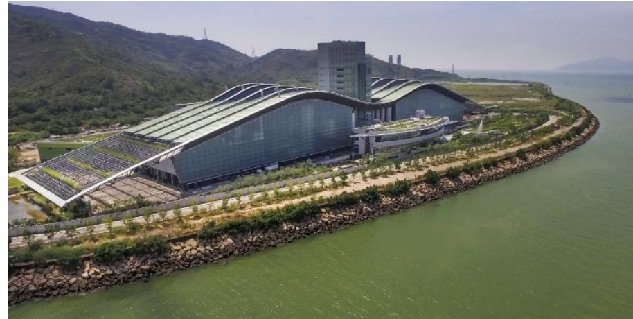
Figure 5.6 T-PARK located at Tsang Tsui, Tuen Mun, has been in operation since April 2015
