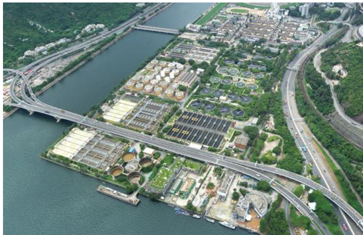
Figure 3.6 Sha Tin Sewage Treatment Works Source: Drainage Services Department
