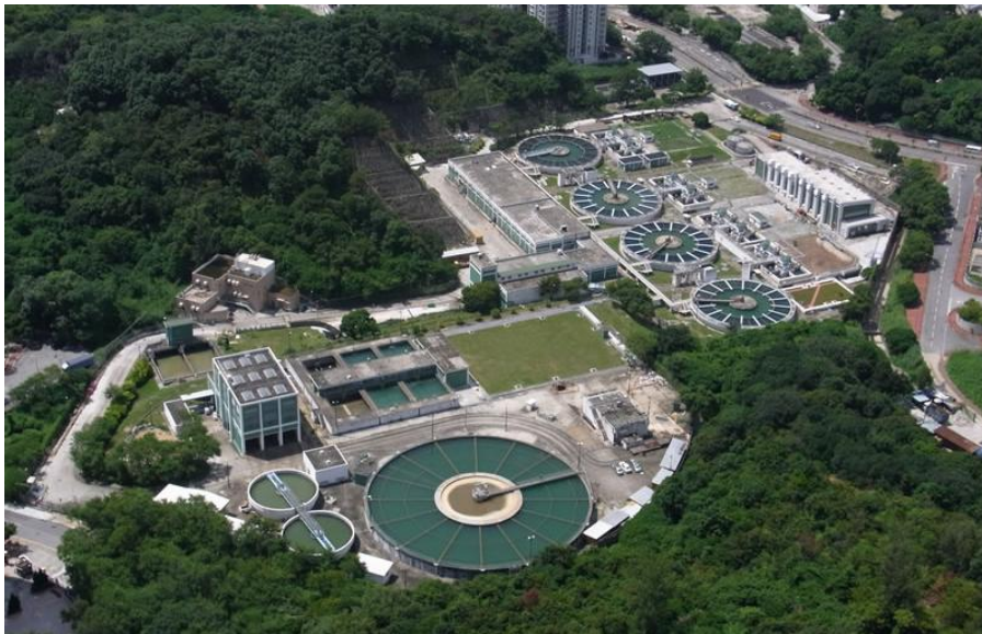
Figure 2.3 Tuen Mun Water Treatment Works
