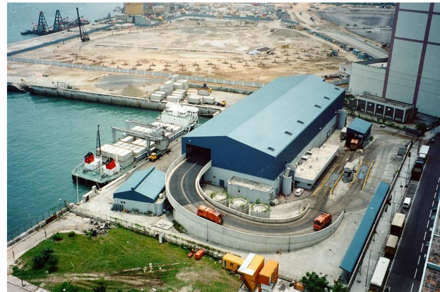
Figure 5.1 Island East Transfer Station
