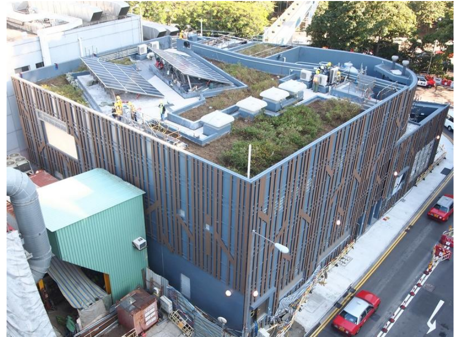
Figure 2.5 New salt water pumping station in Wan Chai
