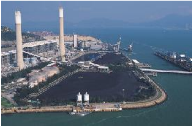
Figure 6.2 Castle Peak Power Station Source: Environmental Protection Department
