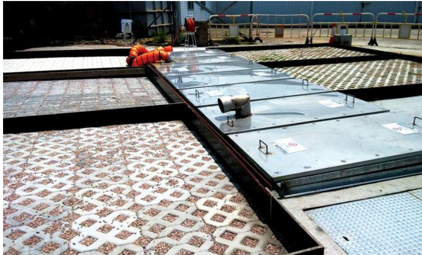
Figure 4.4 Porous pavement in Stonecutters Island Sewage Treatment Works
