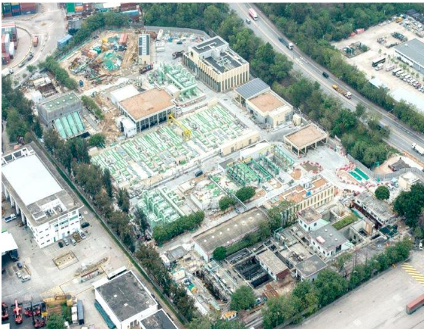
Figure 3.3 Upgraded Pillar Point Sewage Treatment Works Source: Drainage Services Department
