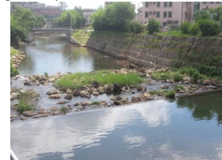
Figure 4.7 Fish ladder built with natural materials at Ho Chung River, Sai Kung Source: Drainage Services Department
